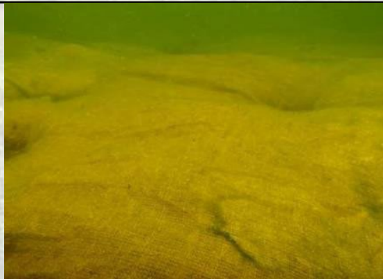
Figure 3 Jute matting secured in situ on the lake bed
