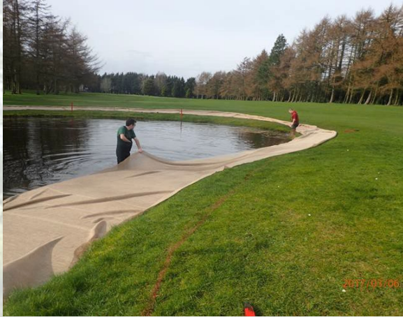
Figures 1&2 Different methods of laying jute matting
