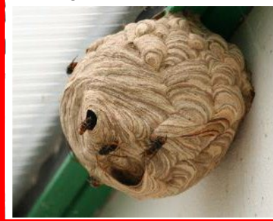
Secondary nest in a building
